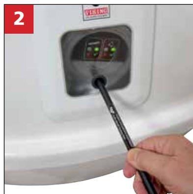
2 Insert testing tool and hold for 5 seconds
